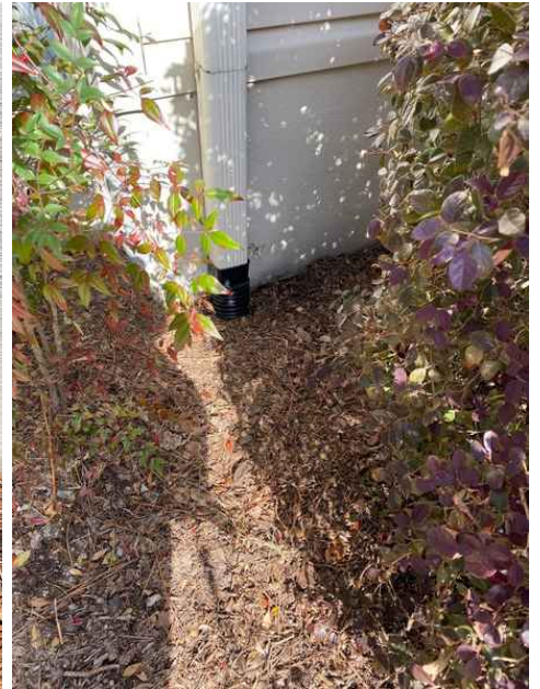
Left front. Was not able to determine end of downspout
